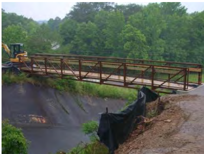
Figure 46 - Bridge installed for crossing Double Oak Lake dam spillway. Source: americantrails.org
